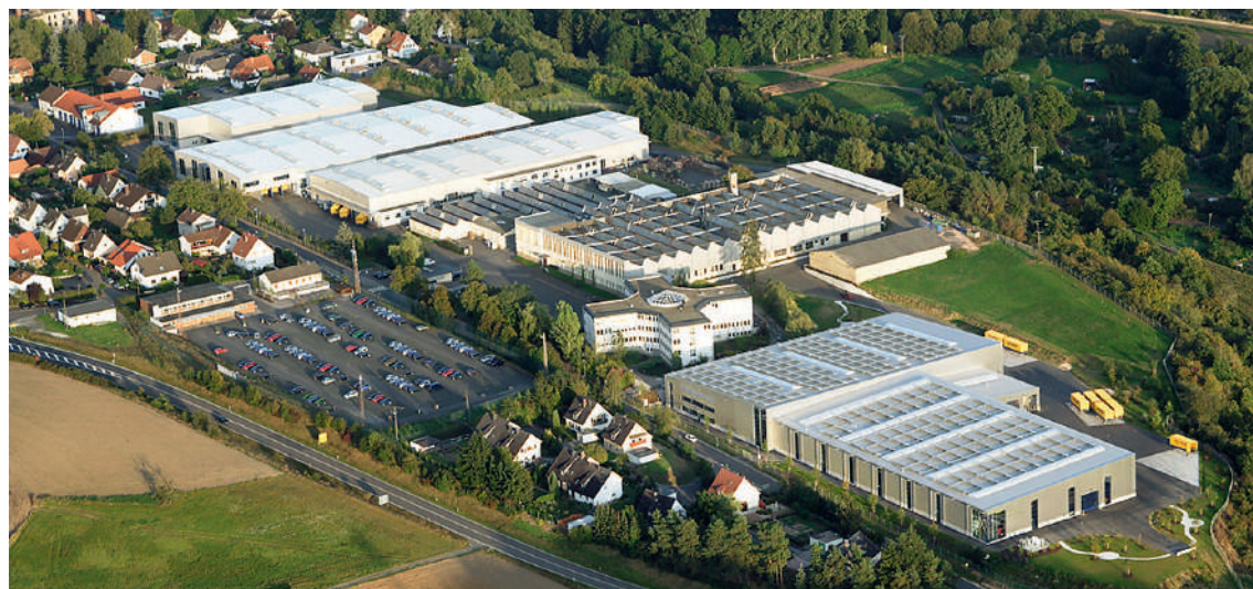
Plant at Meisenheim
