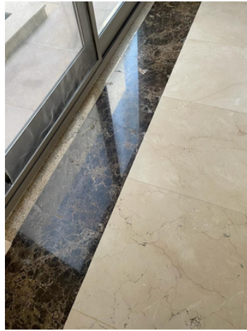
Project: Marble Restoration in Indoor Area of a Villa
