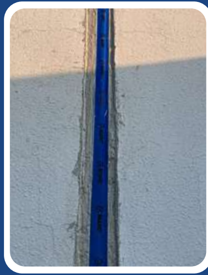
Expansion Joint Treatment
