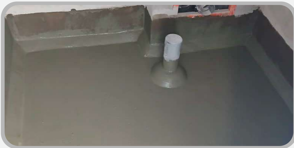
Wet Area Waterproofing
