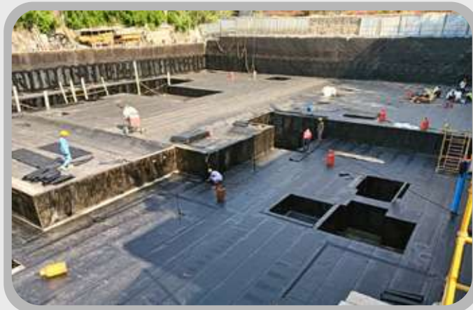
Substructure Waterproofing
