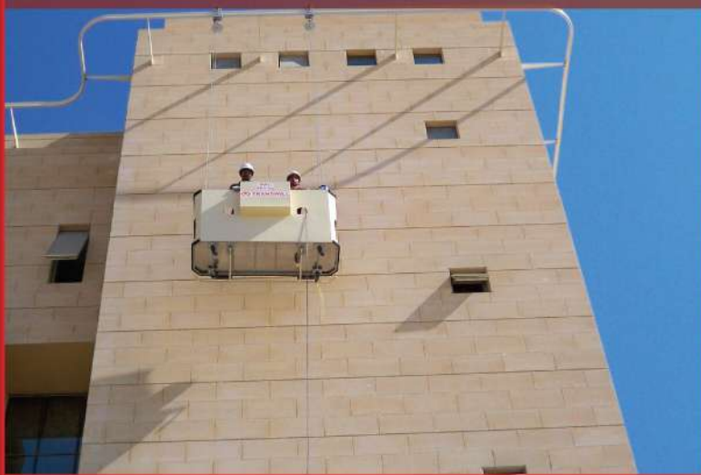
PARAPET TRAVERSING DAVIT
