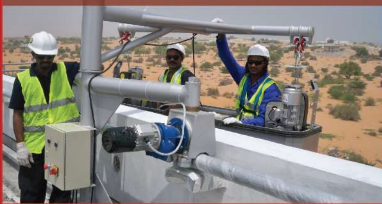
PARAPET MOUNTED DAVIT
