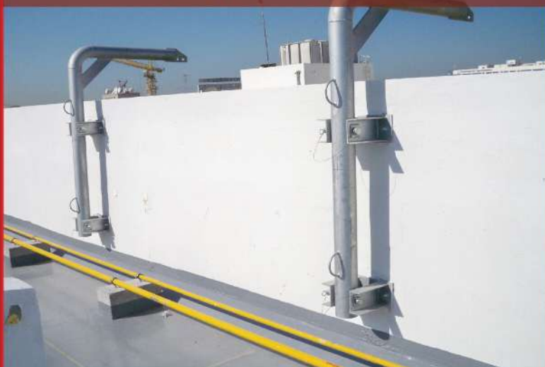
PARAPET MOUNTED DAVIT
