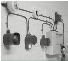
Supply, Installation, Testing and Commissioning
