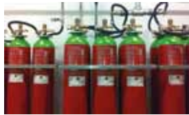
Gaseous Fire Suppression System
