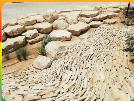
Fixing of Stacking Stones & Laying of Stepping Stones
