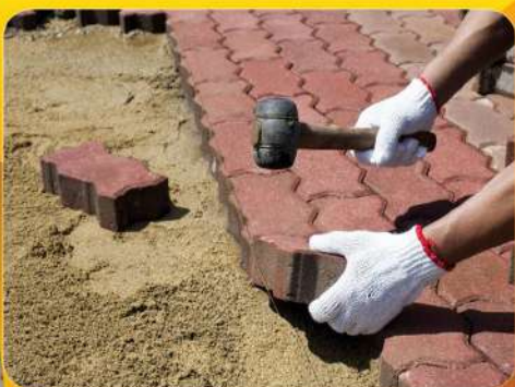
Installation of Interlocks & Concrete Pavers
