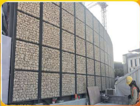
Installation of Gabbion Walls & Retaining Walls
