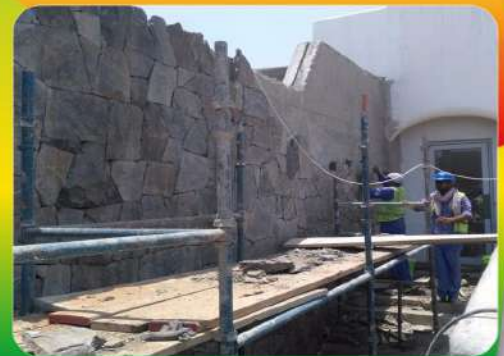
Wall Cladding Rubble stne cladding with Natural Stones
