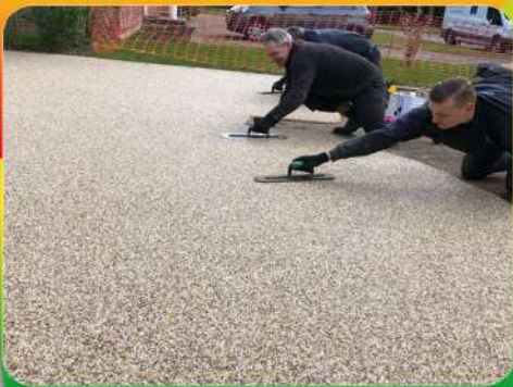
Installation and Compaction of Hogging Path & Resin Pathway
