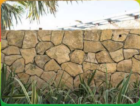
Wall Cladding Rubble stne cladding with Natural Stones
