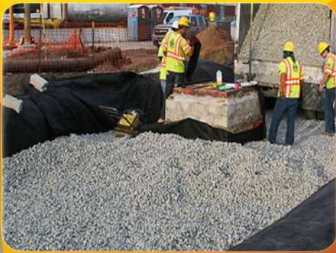
Installation and Laying of Gravels & Road base
