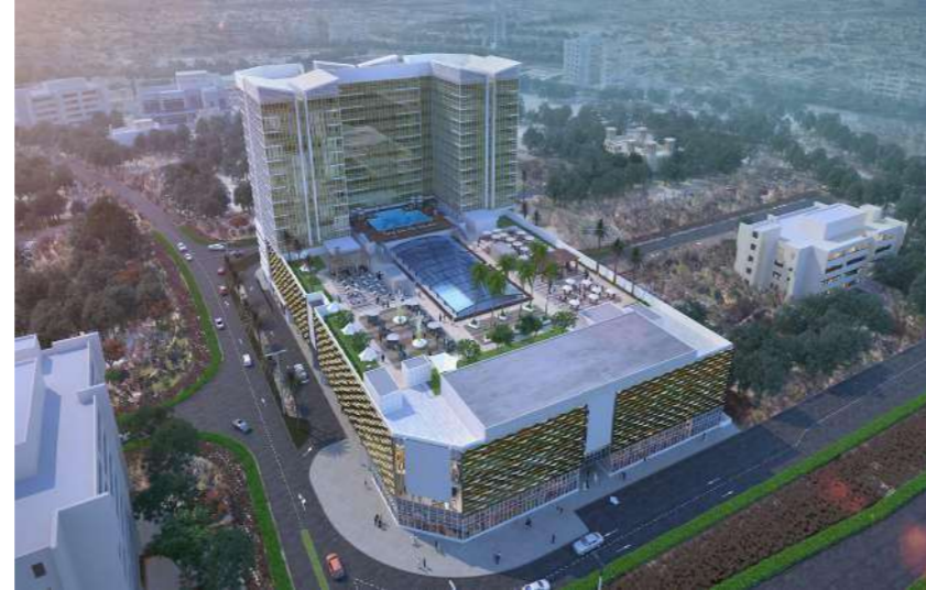
Al Mamzar Byblos Hotel, Guestroom MEP Works
