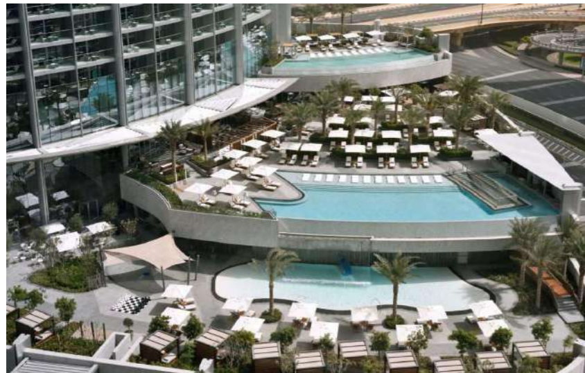
Address Boulevard Hotel Pool & Restaurants MEP
