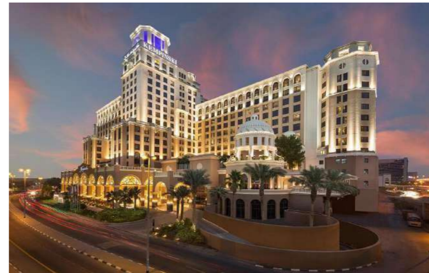
Kempinski Hotel MOE Lightning Protection System
