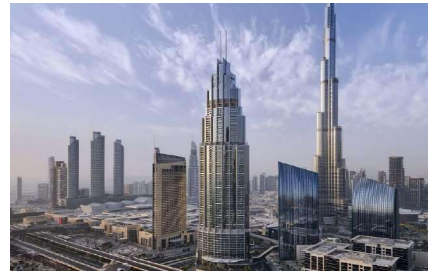
Address Boulevard 11th Floor Luxury Suites Renovation
