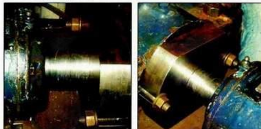
Packing Replaced with Mechanical Seal - After
