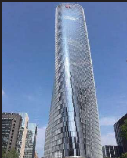
Bank of China Data Center
