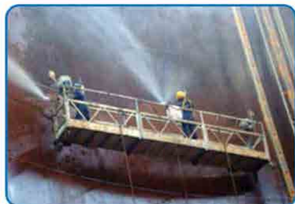
High pressure internal cleaning of tanks
