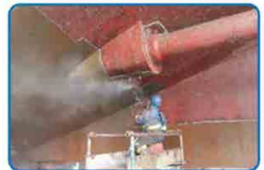
Hydro-blasting of underwater area
