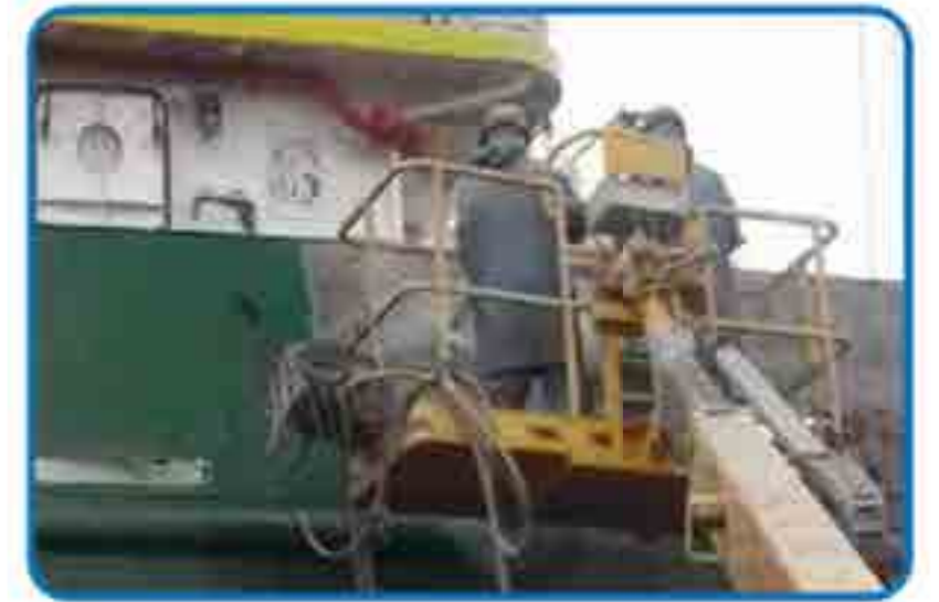
Hydro-blasting of hull area
