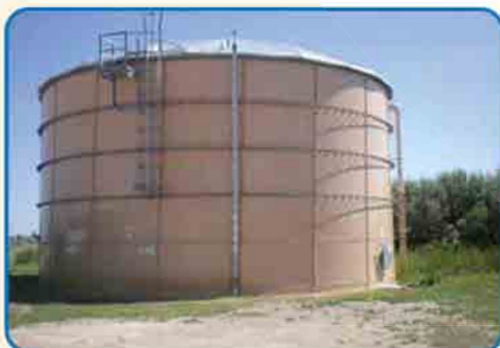
Hydro testing of storage tanks
