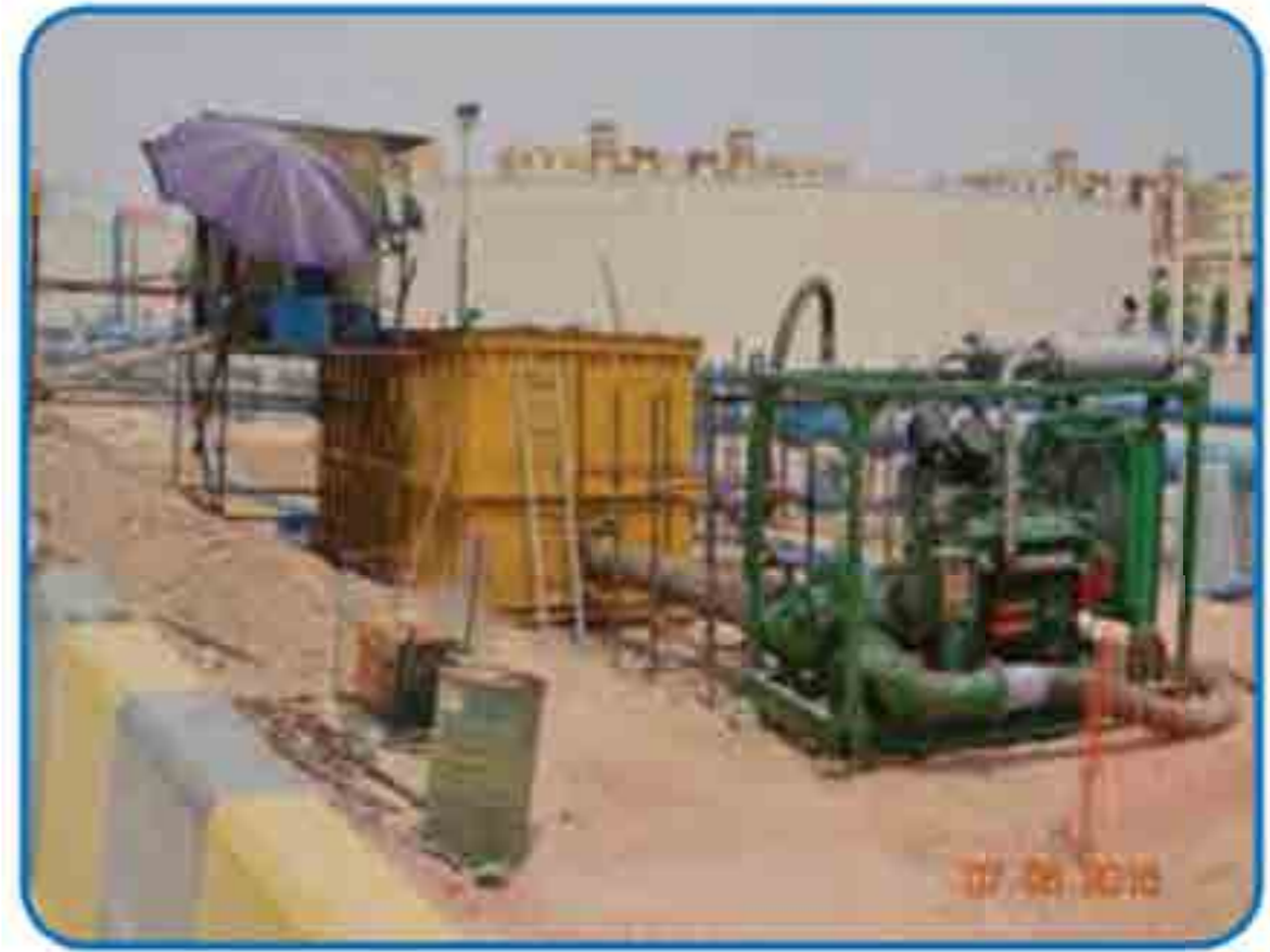
Flushing by open loop system
