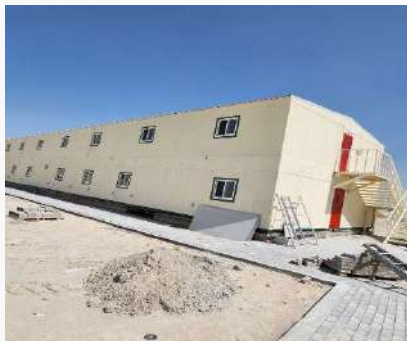
Real Estate Construction Site Site Accommodation Buildings
