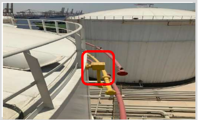
Storage Tank Foam Purer Maintenance
