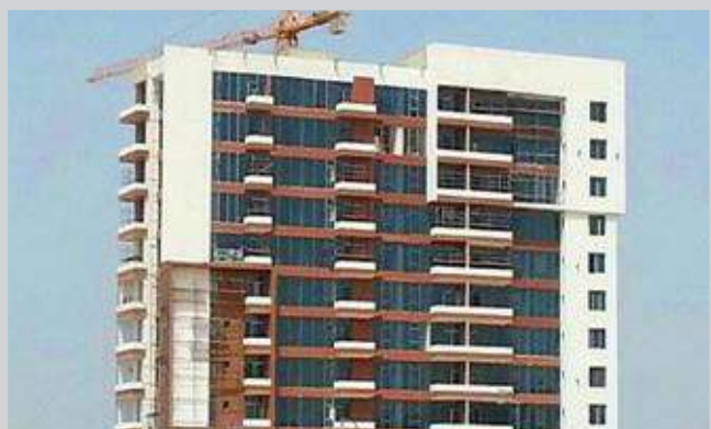
Naresco Contracting, Al Furjan: Full A/ C Works
