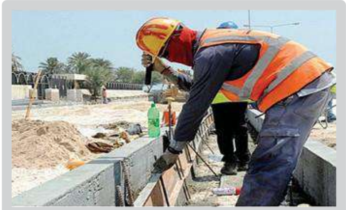
Boundary Wall Work
