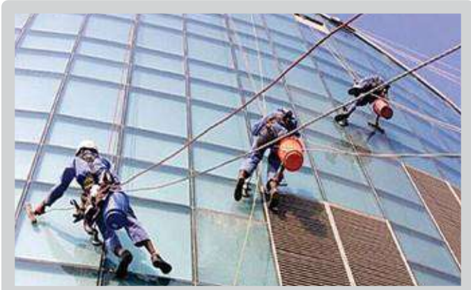
Abu Dhabi: External Light Fixing, Facade Cleaning
