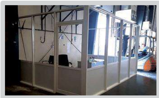
Refurbishment of Office: Aluminum & Glass Partition
