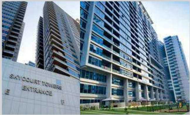
Sky Towers: Facade Cleaning
