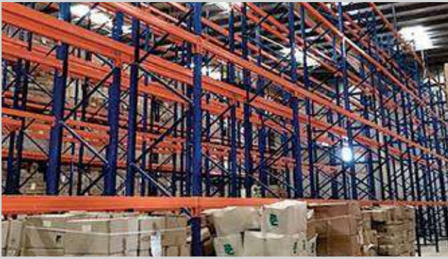
Racking System at a Sharjah Warehouse
