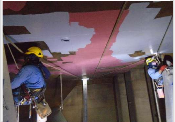
Vessel Tank- Under deck Painting
