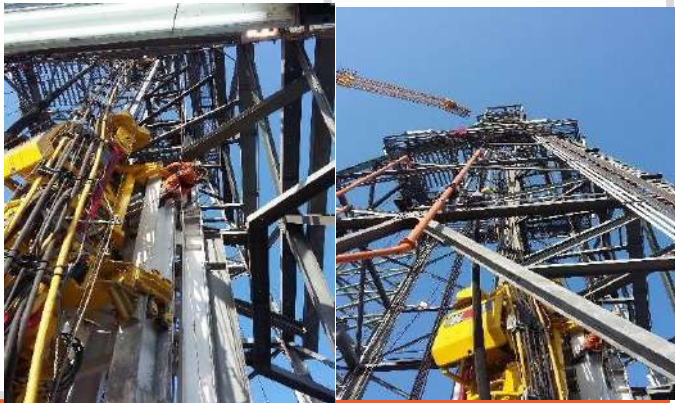
Cable Pulling work
