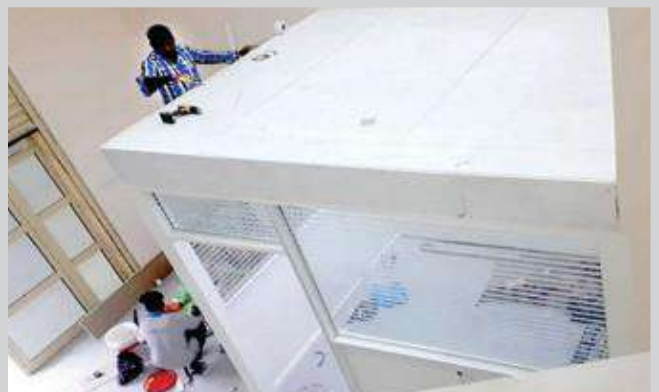
Partition & Renovation of a Warehouse
