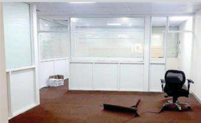
Office Renovation Work
