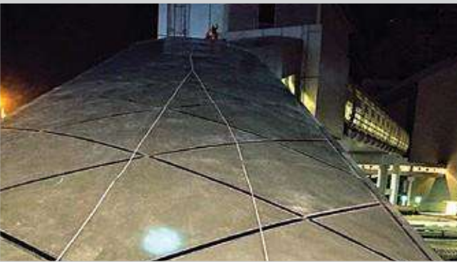
RTA Metro Link Bridge: Facade Cleaning
