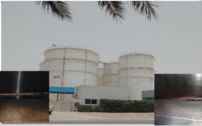
Storage Tank Cleaning
