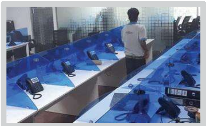
Business Bay Office: Supply & Installation of Work Stations
