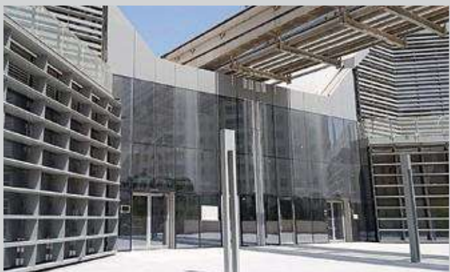
Nakheel Mall: Paving Work
