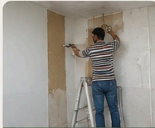
CIVIL & FINISHING WORKS
