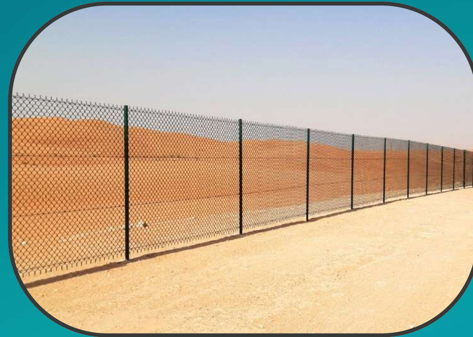
CHAIN LINK FENCE
