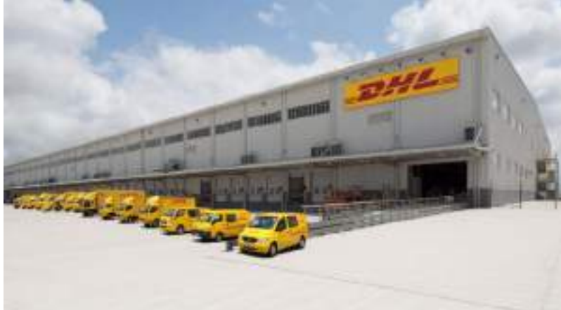
DHL HEAD OFFICE, MEYDAN, DUBAI Cargo Lift ▾
