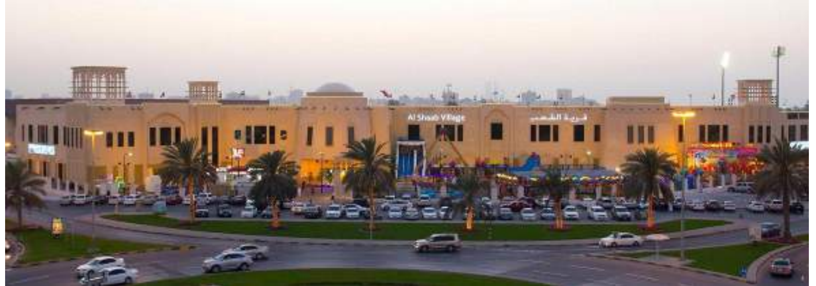
Al-Shaab Village (3 units) MRL, Passenger Lift
