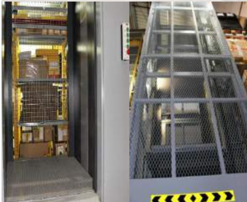
DSV - Global Transport and Logistics Service Lift, 4500 kg, MRL, Freight, 2 stops, 0.5 m/s; Scissor Lift, 2000 Kg ▴
