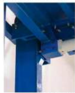
Details of the anti-creep pawl
