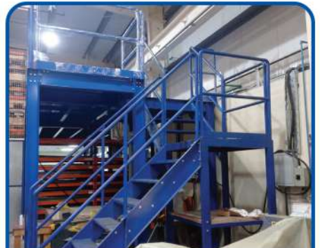
Structural Steel Mezzanine
