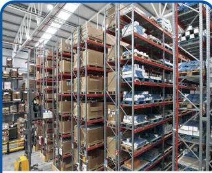
Very Narrow Aisle Racking
