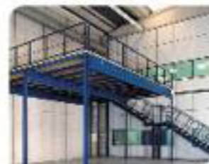
PAINTED MEZZANINE FLOOR
