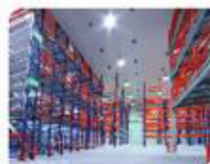
HEAVY DUTY RACK SUPPORTED FLOOR
