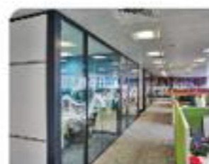
GYPSON & GLASS PARTITION
