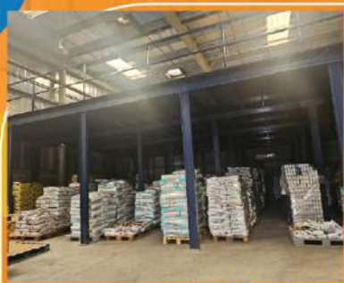
FABRICATED MEZZANINE FLOOR
