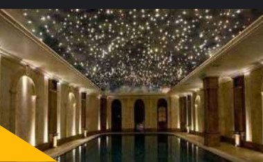
FIBER OPTIC LIGHTING
