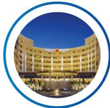
MILLENIUM HOTEL, KSA
