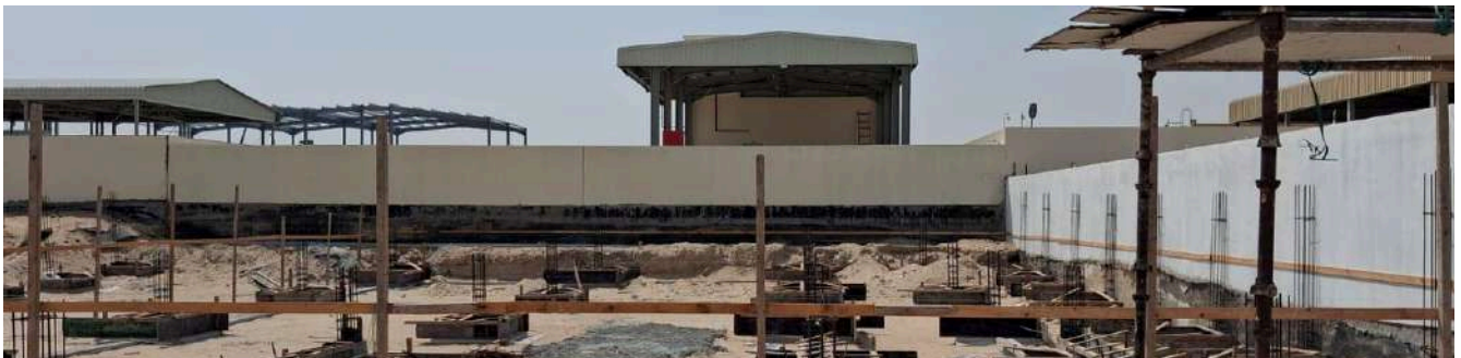
COMPOUND UNDER CONSTRUCTION — SERVICE BLOCK AND SHED FOUNDATIONS
