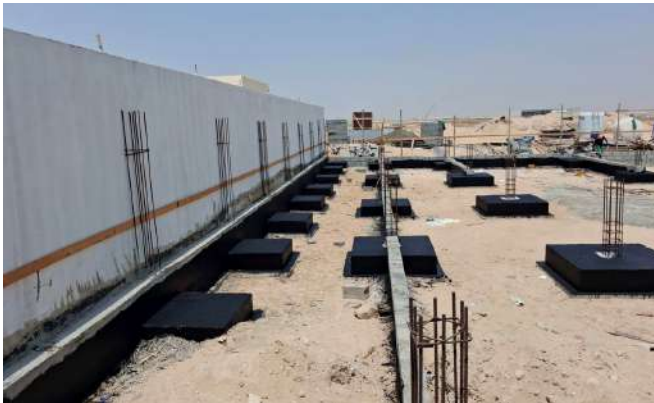
BASES CAST, HOLDING-DOWN BOLTS SET TO SURVEY
