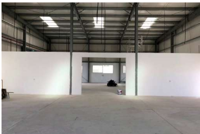
SERVICE BLOCK PARTITION AND GLAZING
