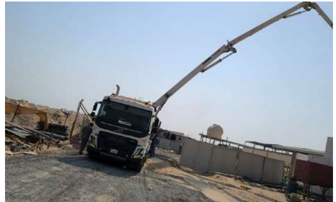
CONCRETE PLACEMENT BY BOOM PUMP
