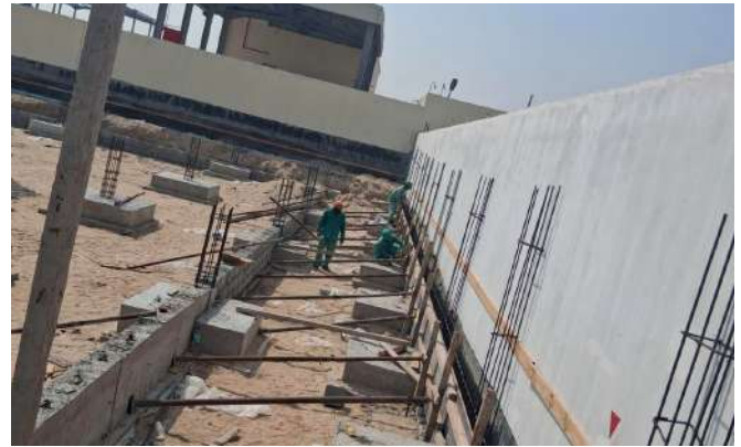
BOUNDARY WALL AND COLUMN STARTER BARS
