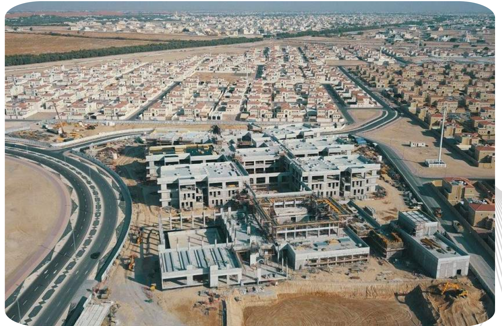
Infrastructure Construction Project Abu Dhabi
