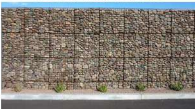
Gabion wall materials
