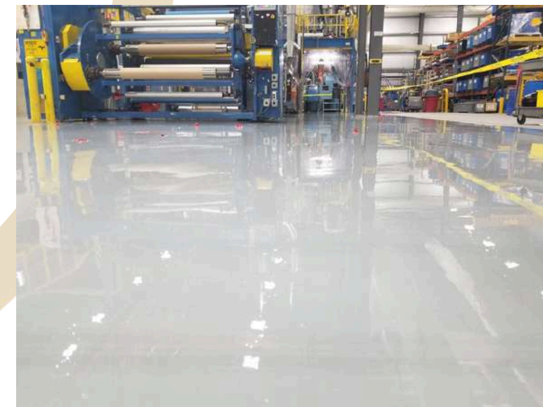
Epoxy Flooring System
