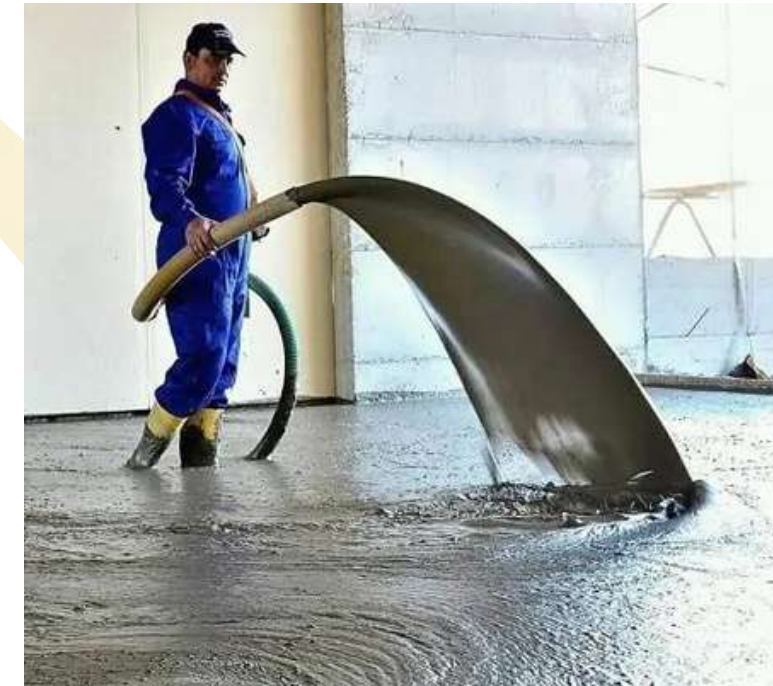
Foam Concrete & Concrete Repair
