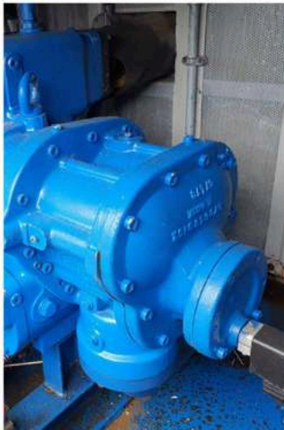
7. Chiller Compressor Overhauling Work
