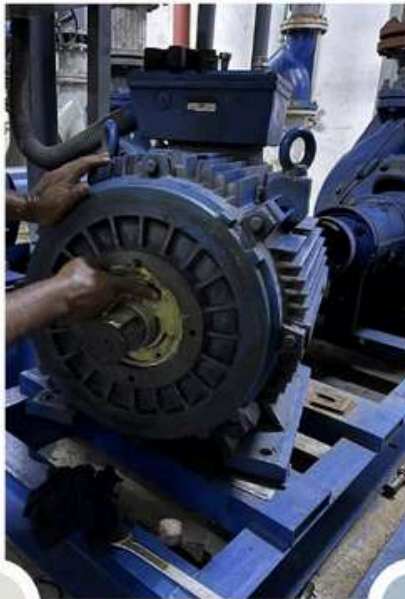
2. Chiller Water Pump & Motor Maintenance.
