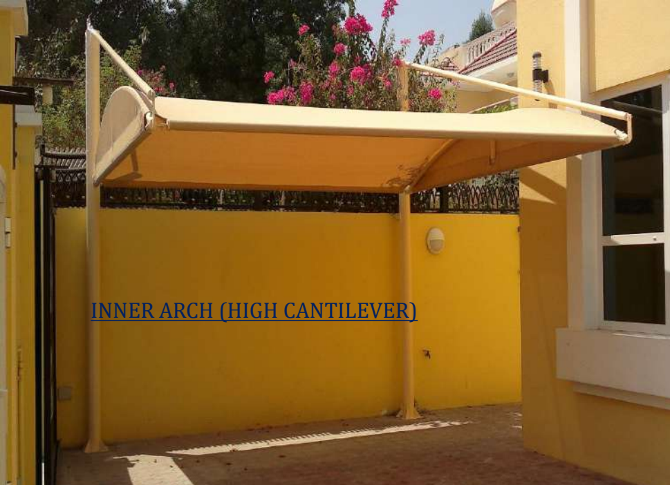
INNER ARCH (HIGH CANTILEVER)
