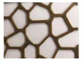
The designers wanted to incorporate elements of the sea in the architecture. Prime Metal Craft used their design to create a thick metal mesh that emulates coral and stone for an organic and simple design.
