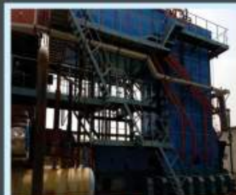
Gharibsons Karachi, Coal Conversion of 50 TPH steam boiler
