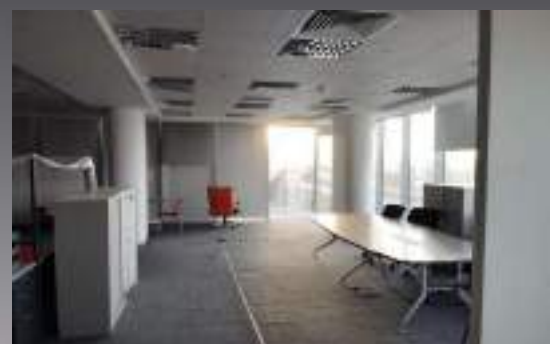
HASSANICOR COMMERCIAL BUILDING OFFICES MODIFICATION, AL BARSHA
