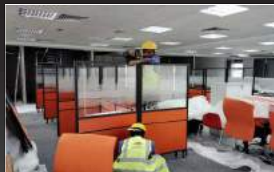
HASSANICOR COMMERCIAL BUILDING OFFICES MODIFICATION, AL BARSHA
