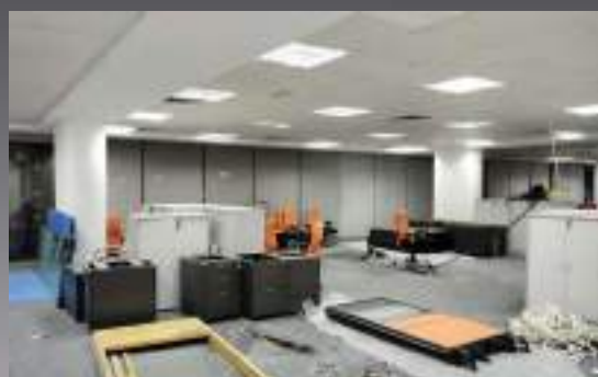
HASSANICOR COMMERCIAL BUILDING OFFICES MODIFICATION, AL BARSHA
