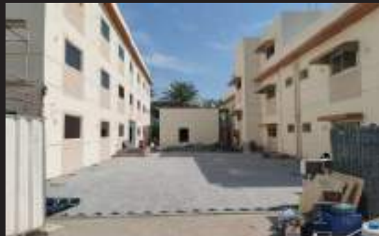
LADIES STAFF ACCOMODATION - G+2+R - CROWN PRINCE PALACE - FUJAIRAH
