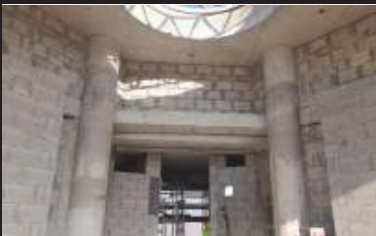
CONSTRUCTION OF CHALETS - BAB AL SHAMS DESERT RESORT - AL QUDRA
