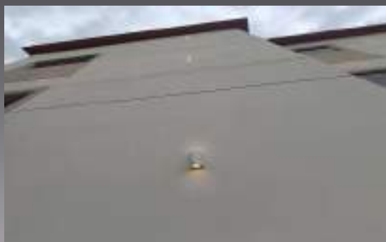
LADIES STAFF ACCOMODATION - G+2+R - CROWN PRINCE PALACE FUJAIRAH
