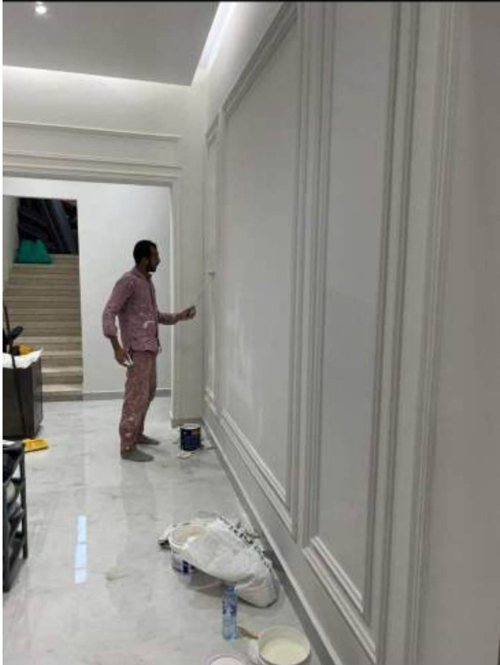
Molding and paint work
