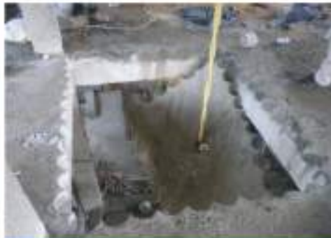
CONCRETE SLAB CUTTING
