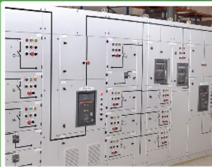
Low Voltage Switch gear Panel
