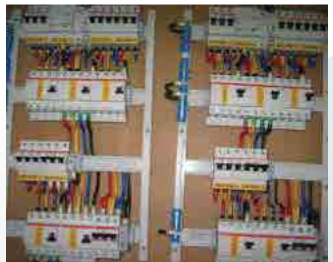
Final Distribution Board (Internal View)
