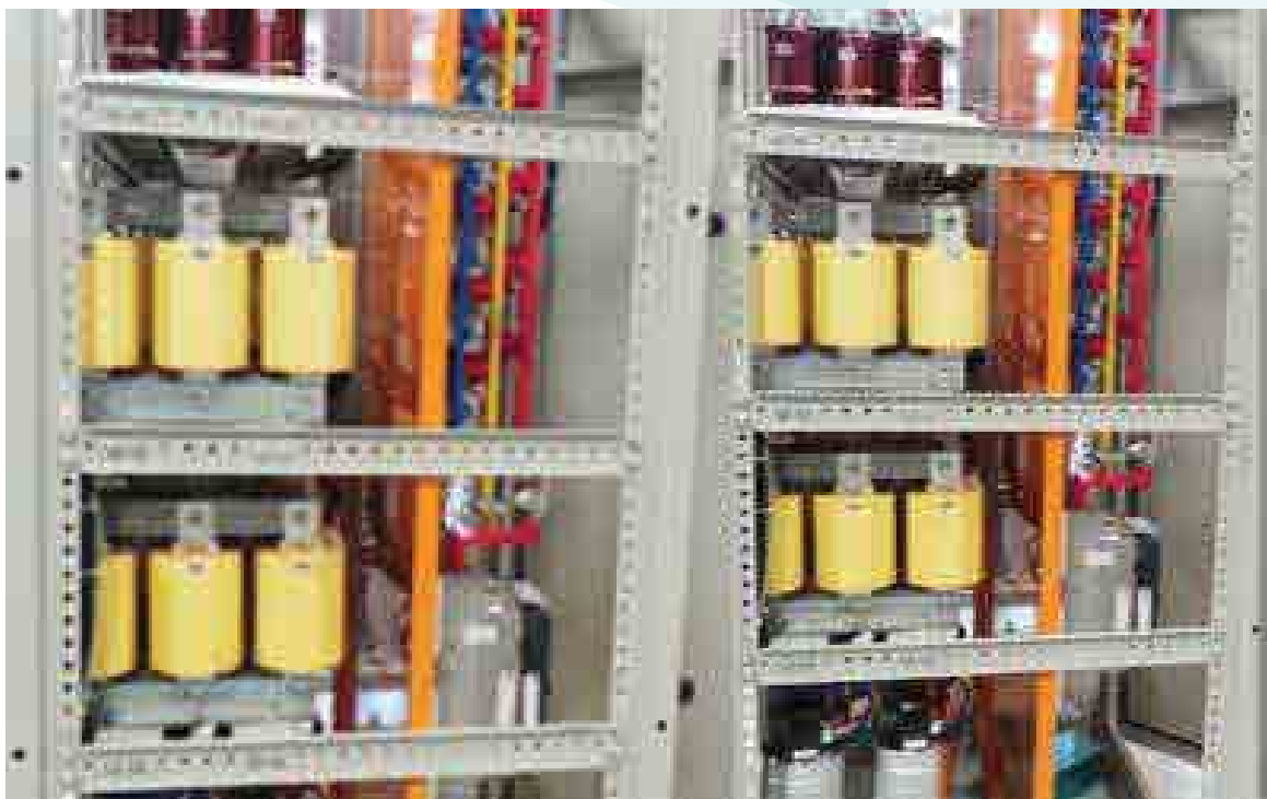
400KVAR Capacitor Bank with Harmonic Filter (Detuned Reactor)
