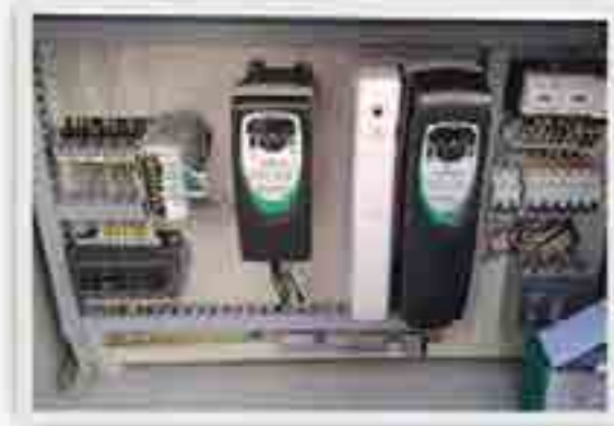
VFD CONTROL PANELS
