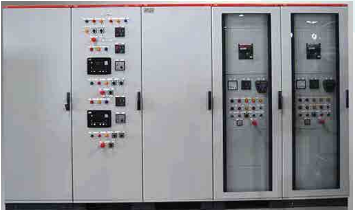
4 Generator Synchronizing panel
