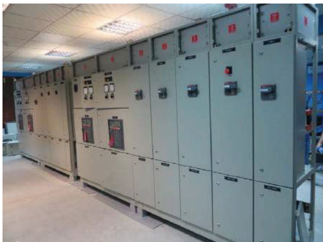
PANEL REFERENCE : 2500A LV PANEL PROJECT : NATIONAL STORE CONTRACTOR : SAM BUILDING MATERIALS
