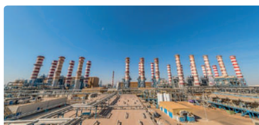
QATAR ELECTRICITY & WATER TOWER
