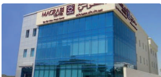
MAGRIBI CENTER PROJECT
