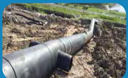
A typical landfill uses leachate collection systems to protect the water and the environment from landfill contaminants. These systems use a series of high-density polyethylene riser shafts, which must have additional pipe continuously added to the riser as the landfill soil cover increases in height. The characteristics of HDPE pipe and fittings allow these systems to be continuously modified as the landfill progresses.
