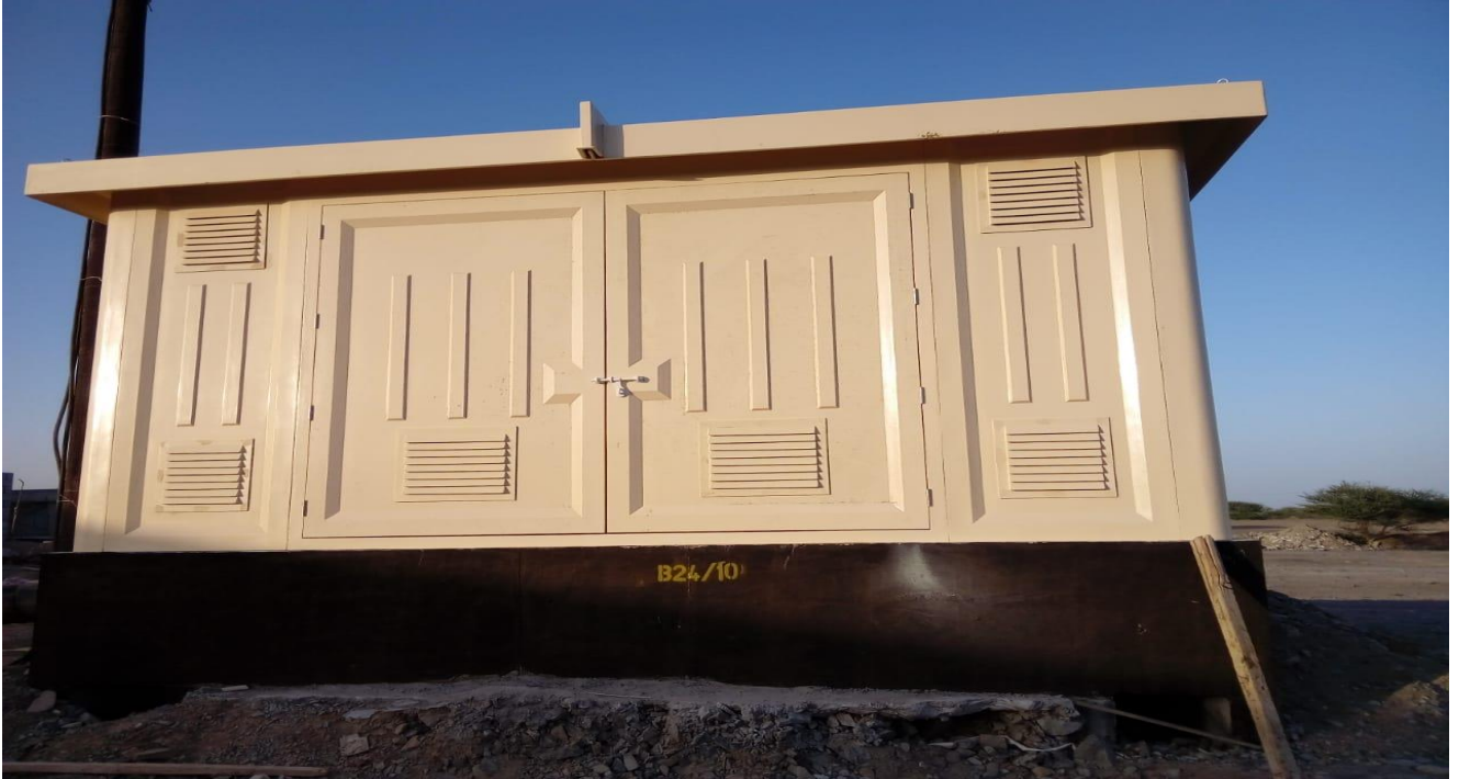
GRP TRANSFORMER ENCLOSURE
