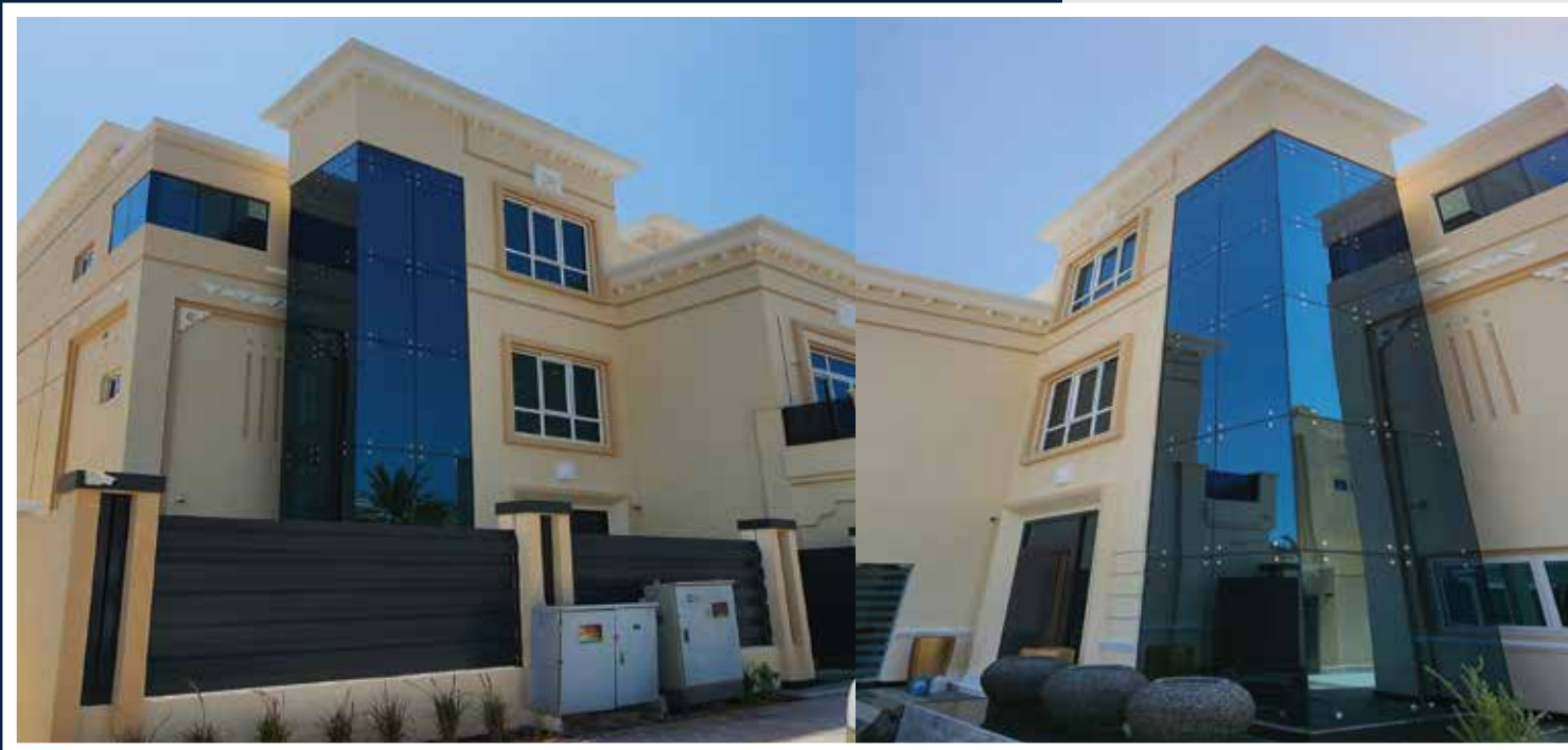
MARINA VILLA -99 CLIENT-ARAB EMIRATES SCOPE OF WORK : LIFT AREA GLASS WORK ( WITH SPIDER) AND CLADDING
