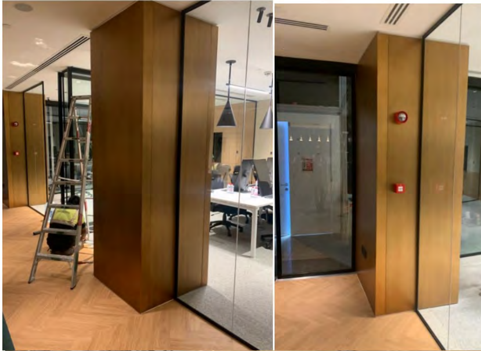
STAINLESS STEEL CLADDING WORKS- PMO OFFICE
