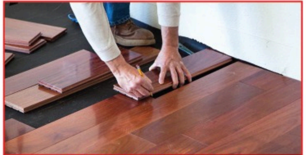
FLOOR REPAIRS & FITTING
