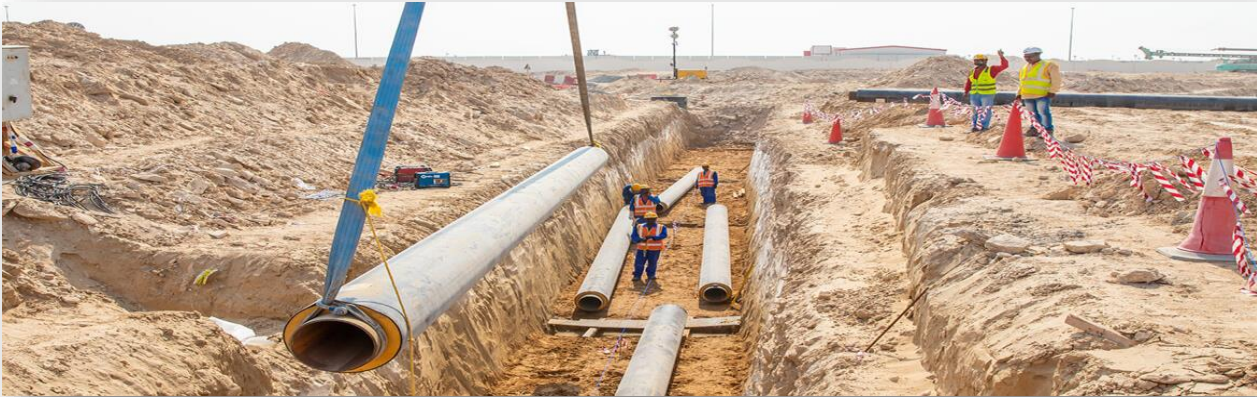
DRAINAGE WATER PIPE INSTALLATION
