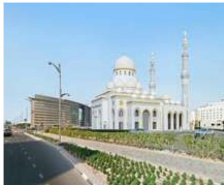
Construction of HHS Rashid Bin Mohammed Mosque in Hudaiba, Dubai
