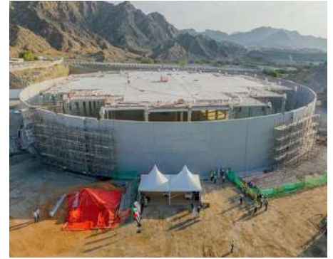
DEWA – Construction of 30 MIG Water Reservoir in Hatta
