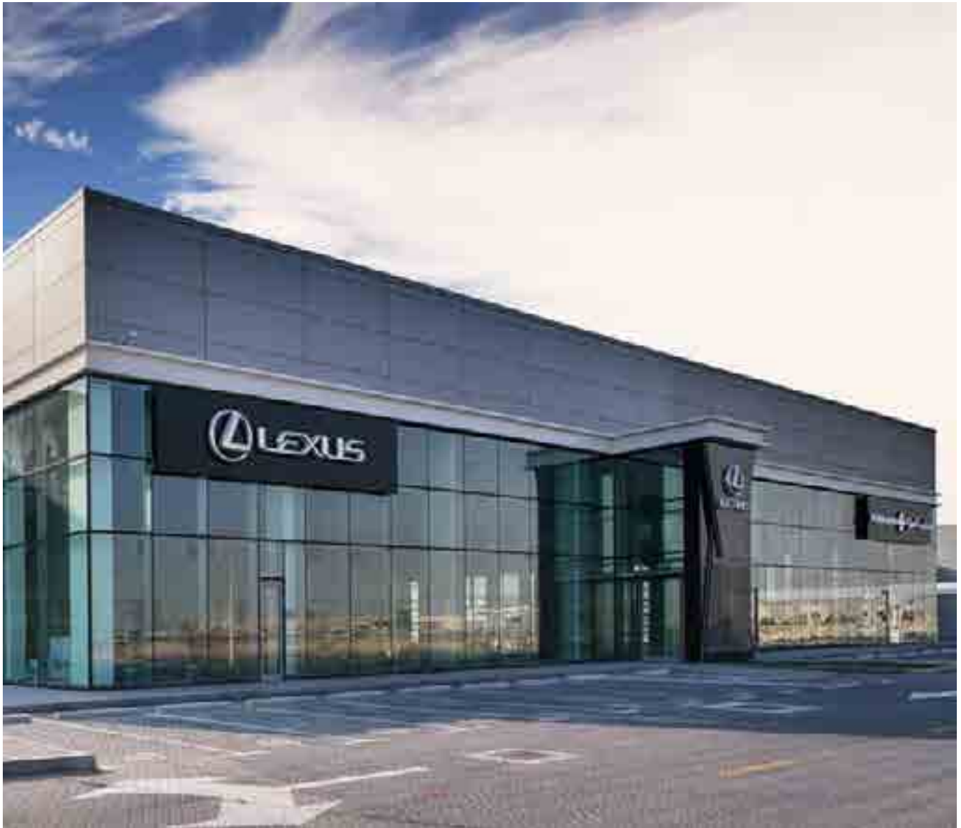
AL FUTTAIM GROUP – TOYOTA & LEXUS SHOW ROOM – EPOXY FLOORING AND CAR PARK COATING
