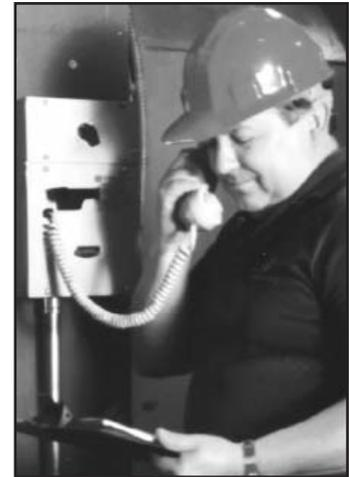
The GAI-Tronics Page/Party® System is a distributed amplifier system. Each indoor, outdoor, or hazardous area wall station contains a power amplifier for driving speakers. This configuration offers a major advantage: when an amplifier is removed, only the associated speaker is inoperable; all other system speakers will continue to broadcast pages.
