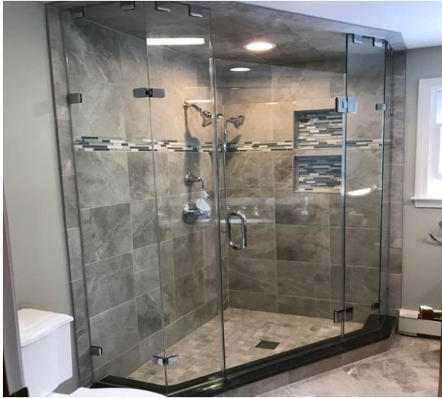
Full height glass shower cubicles.
