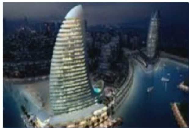
Project Name: Sail Tower Company Name: Al Rakha General Contracting LLC Location: Abu Dubai, UAE
