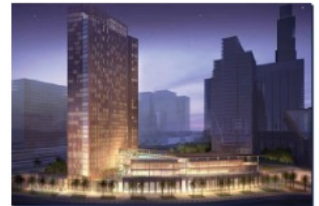
Project: Four Season Hotel Work: Painting. Main Contractor: Al Futtaim Carillion LLC. Location: Al MaryahIsland, Abu Dhabi.
