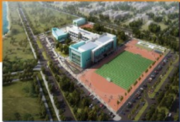
Project: Amity International School Company Name: ShapoorjiPallonji Mideast LLC. Location: Al Bahya, Abu Dhabi, UAE Starting Date: March-2014
