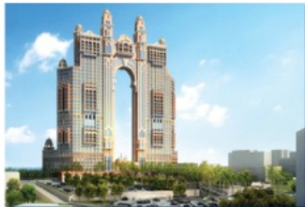
Project: Fairmont Hotel & Service Apartments. Main Contractor: Depa Décor General Contracting & maintenance Co LLC. Location: Marina Mall, Abu Dhabi.
