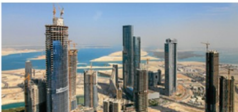
Project: City of Lights Company Name: China State Construction Engineering Corporation (Middle East) LLC Location: Al Reem Island, Abu Dhabi, UAE.
