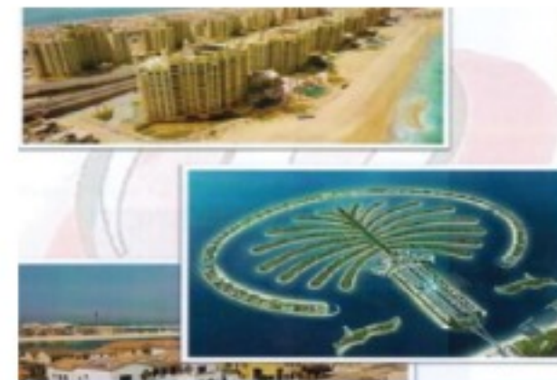
Project Name: Palm Jumeirah Company Name: Al Gaith Construction Company Location: Dubai, UAE.
