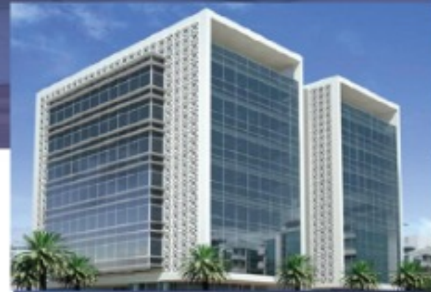
Project Name: Sorouh North Park Office Building Company Name: Orient House for Development and Construction Co. LLC. Location: Abu Dhabi, UAE
