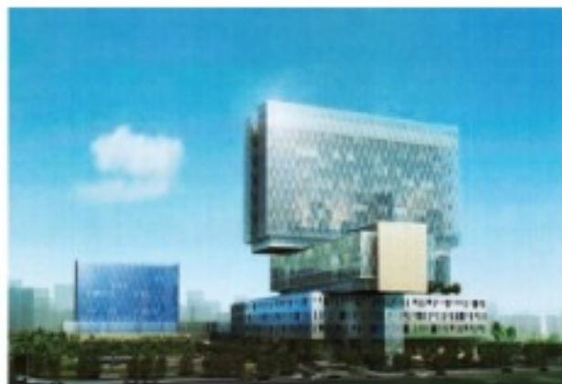
Project: Cleveland Clinic Company Name: Six Construct Co Ltd. Location: Abu Dhabi, UAE.
