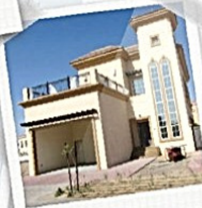
G+1 RESIDENTIAL VILLA FOR PRIVATE OWNER IN "THE VILLA" @ DUBAI LAND ON PLOT RO-017
