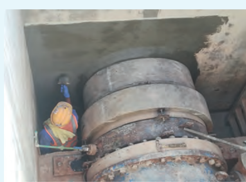
Injection works in Under-ground Pipe Chamber
