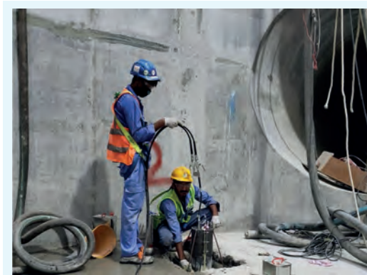
Sealing of De-watering Wells
