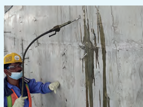
Crack Injection
