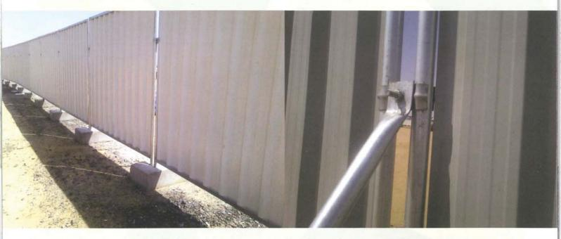
Corrugated sheet fence standard height is 2.4 meters mounted height and there are two types of fence usually made. One is panel type and another is continuous type without any gap in between. These fences are installed at site with concrete blocks of different sizes above the ground.
