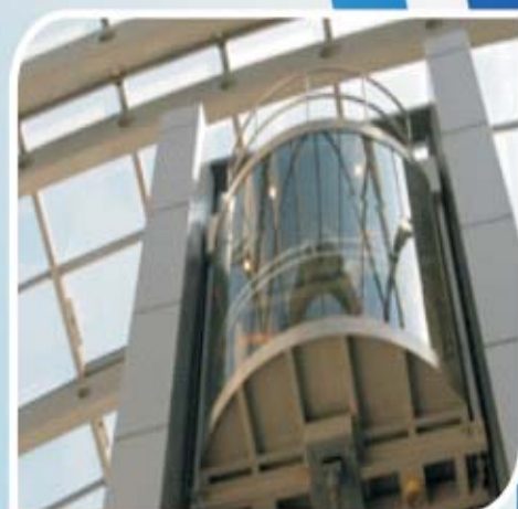
Outside mounted glass elevator
